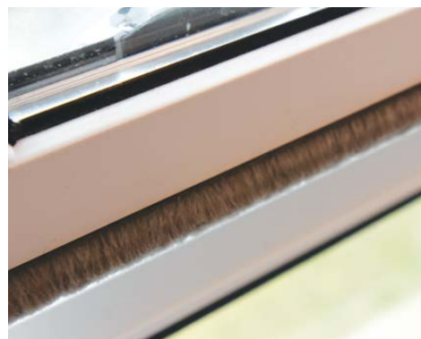
Triple weather stripping
